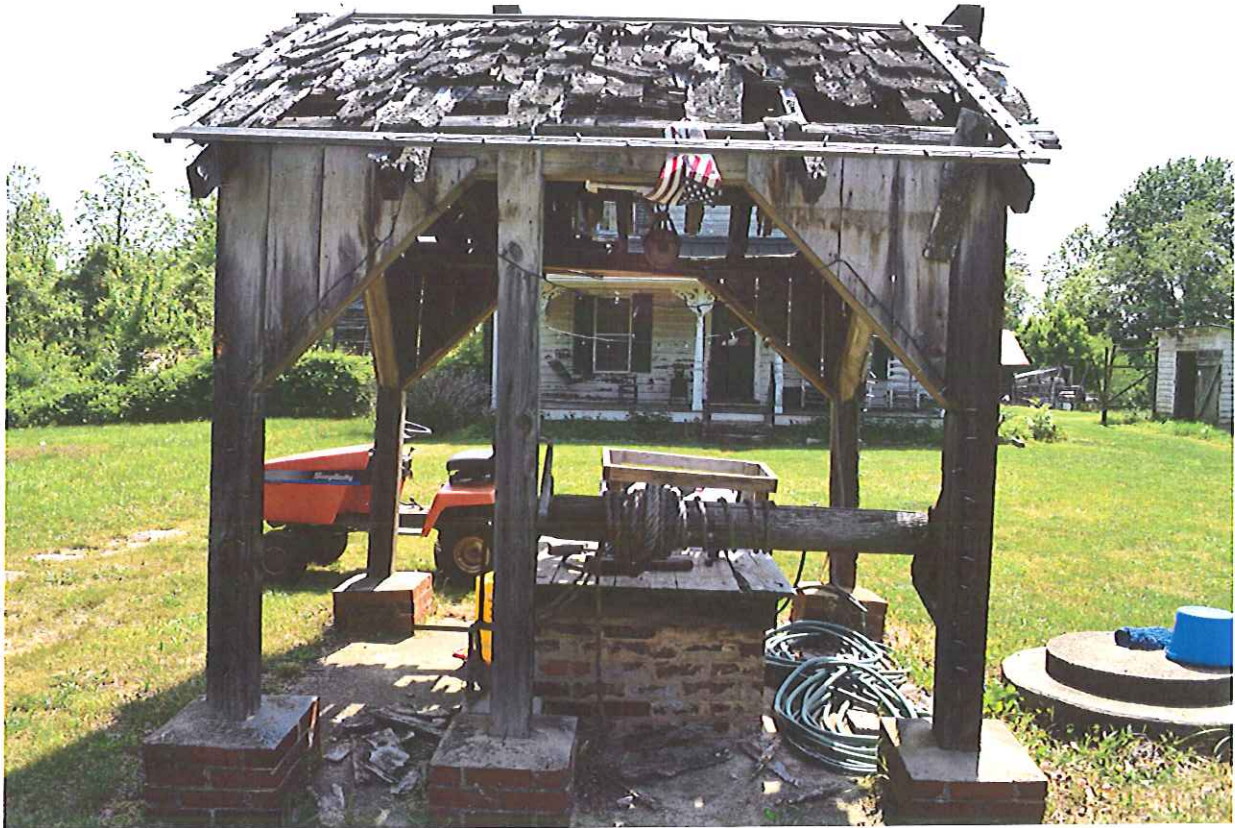
Figure 19: Well and well house, facing east
