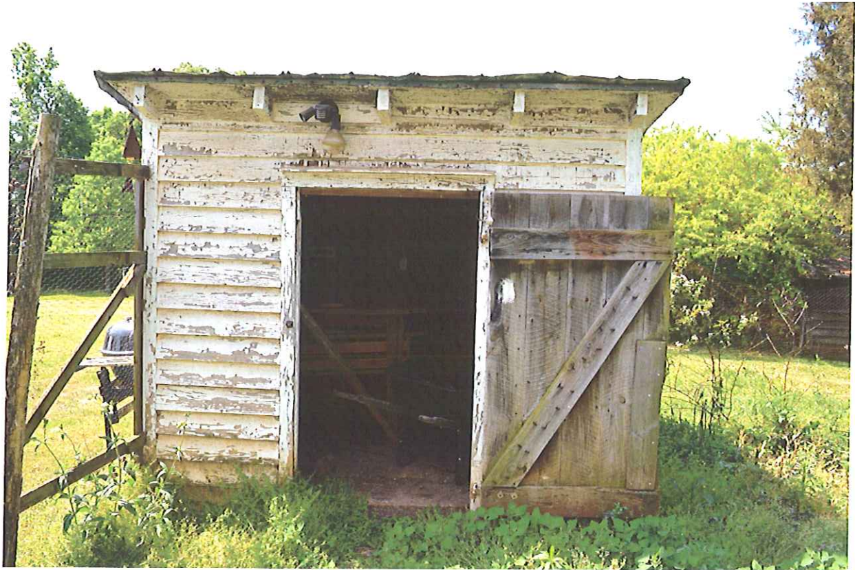
Figure 18: Generator building, facing south
