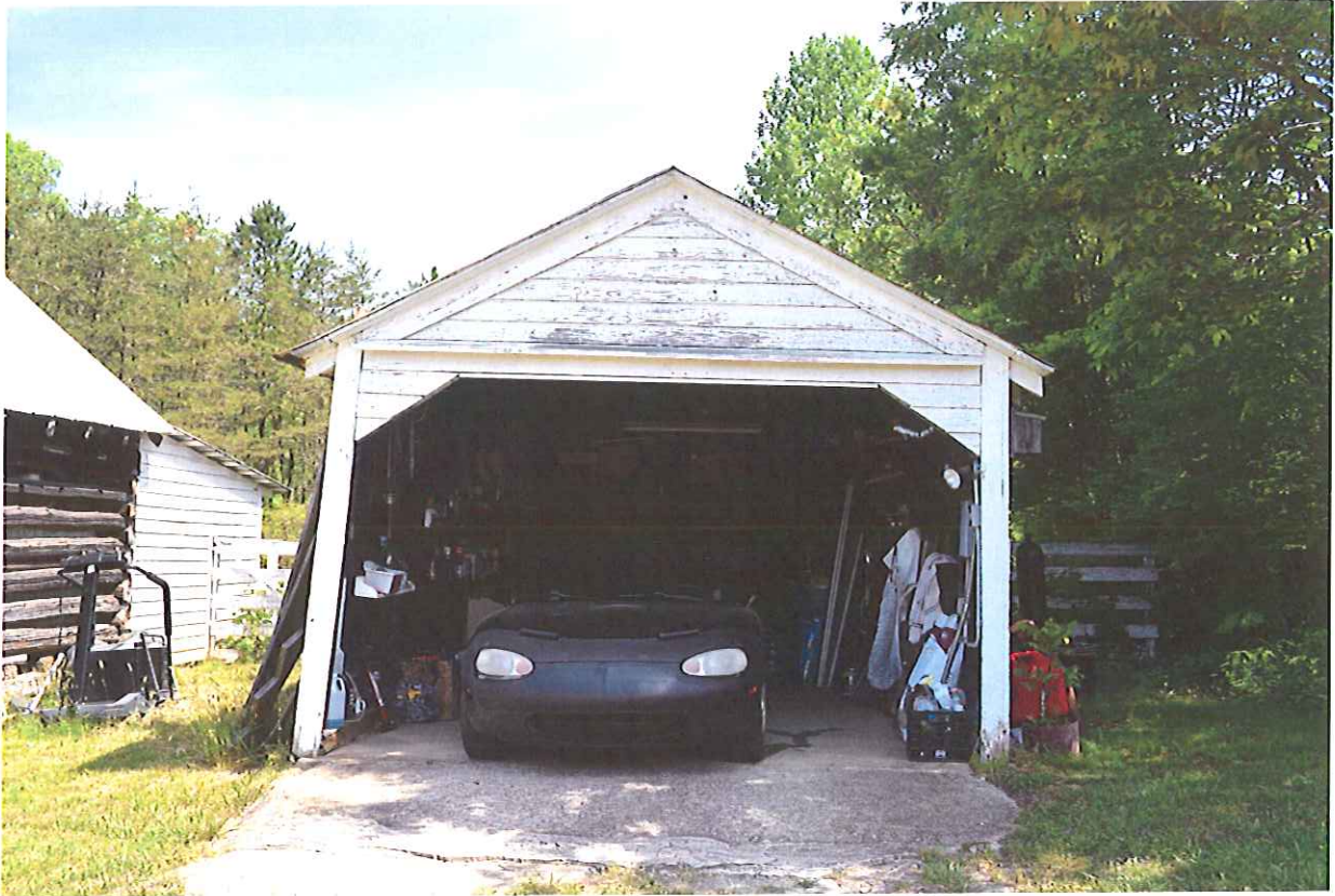
Figure 11: South elevation of the garage, facing north
