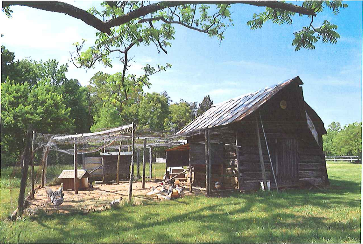
Figure 16: Northeast corner of smokehouse, facing southwest
