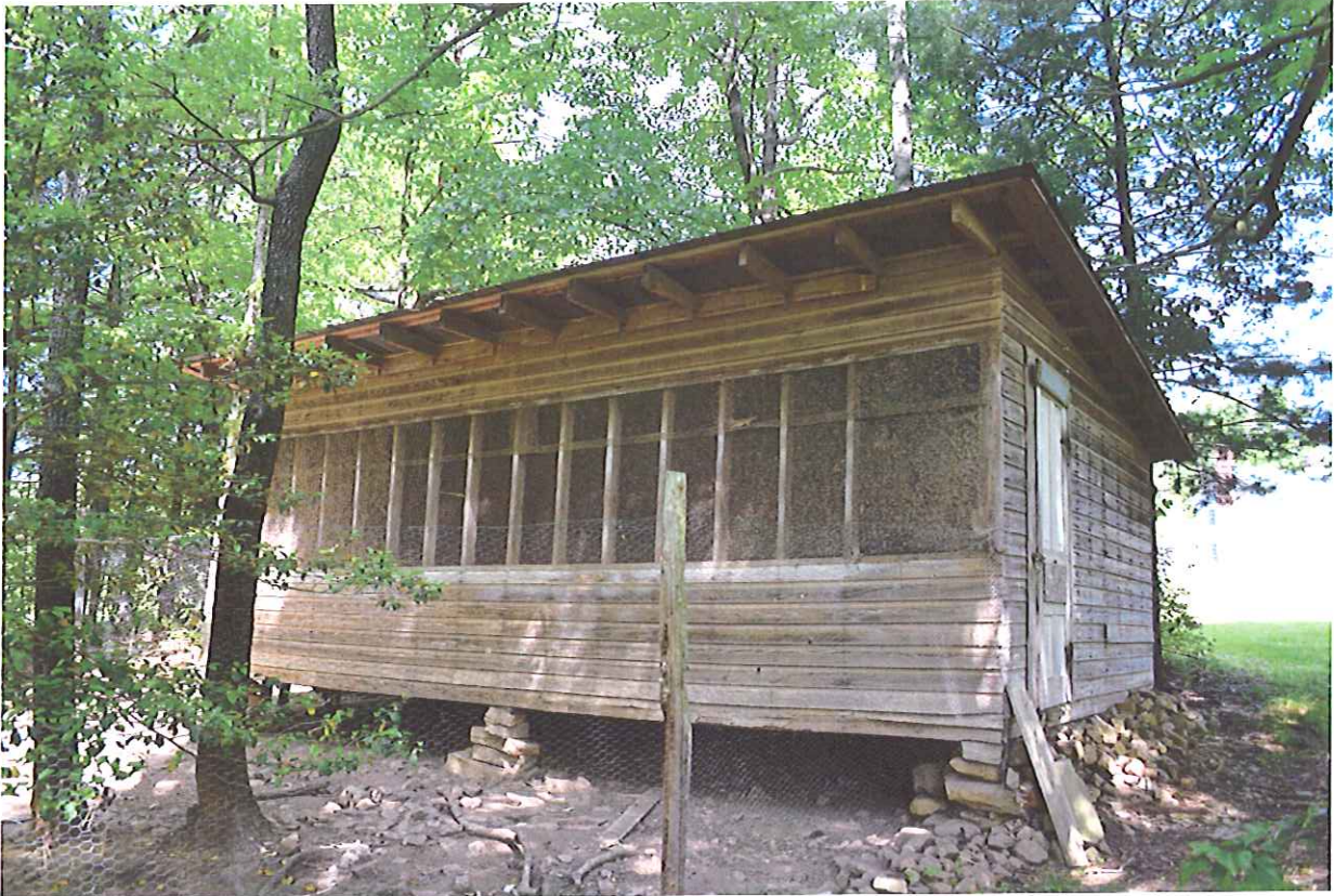
Figure 17: South elevation of the chicken house, facing north-northwest
